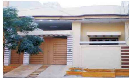
A single-storeyed house
