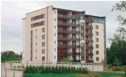
A block of flats
